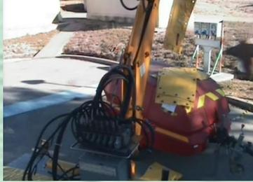
Placing lead mattresses on an irradiated and contaminated module
